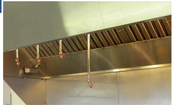
*The nozzles above the cooking equipment spray wet chemicals once any smoke or grease-laden vapor is detected.*
