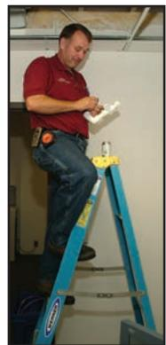
*Workers should not step on top cap of a step ladder.*
