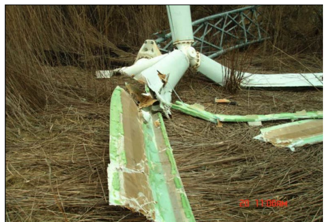
A wind turbine tower collapsed because the turbine blades became unbalanced when one of its blade weights fell off.
