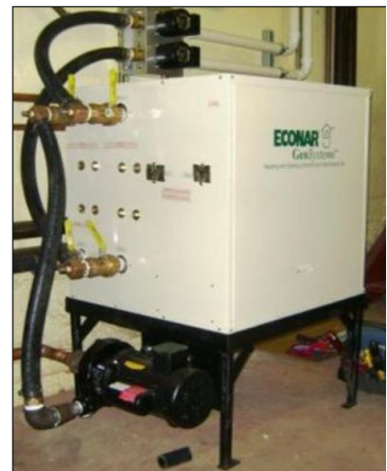
Ground-source heat pump
