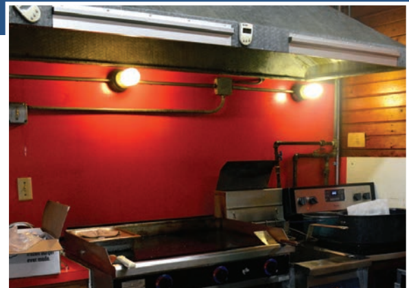
Train employees about how to remove grease and oil sludge.
