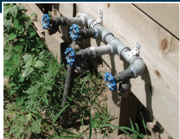
Backflow preventers can be used to keep water from flowing back into the water source.
