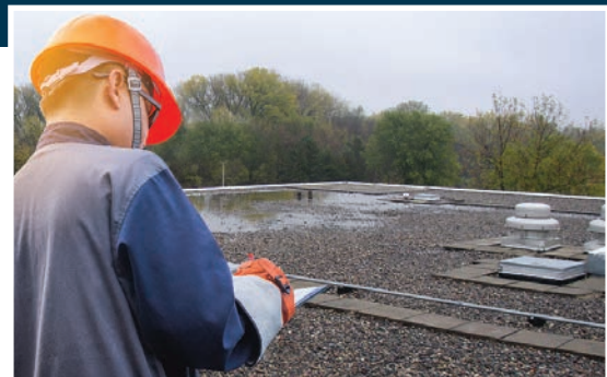
Routine inspections are essential in preventing unplanned problems.
