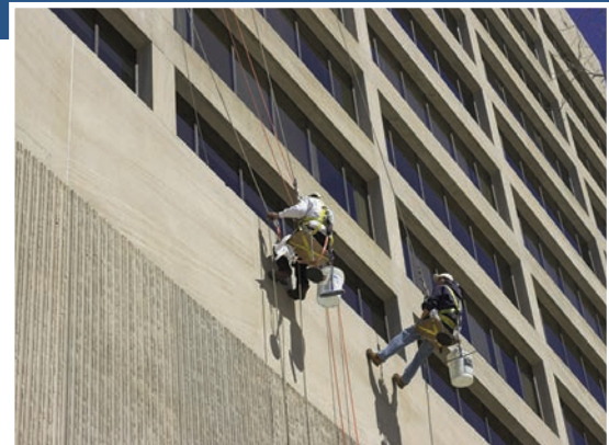
Window washers use rope descent safety system.
