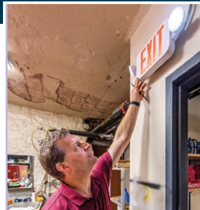
Emergency lighting must be tested monthly and yearly.
