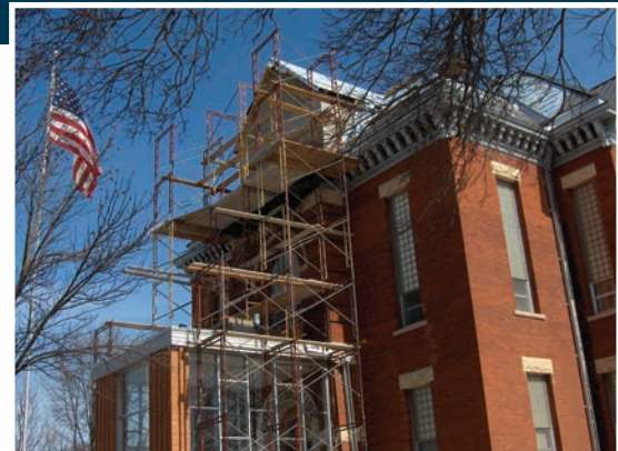
Document any rooftop repairs as part of a roof management program.
