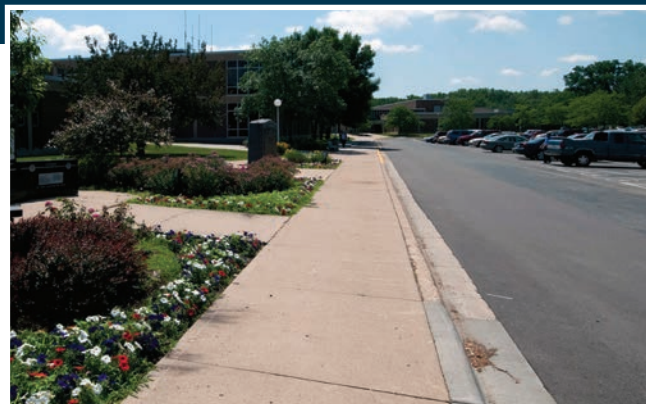
Periodically conduct inspections of outdoor walking surfaces.
